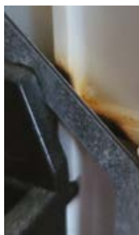
↑ The earth strap on the back of the shower isolator had been getting very hot
